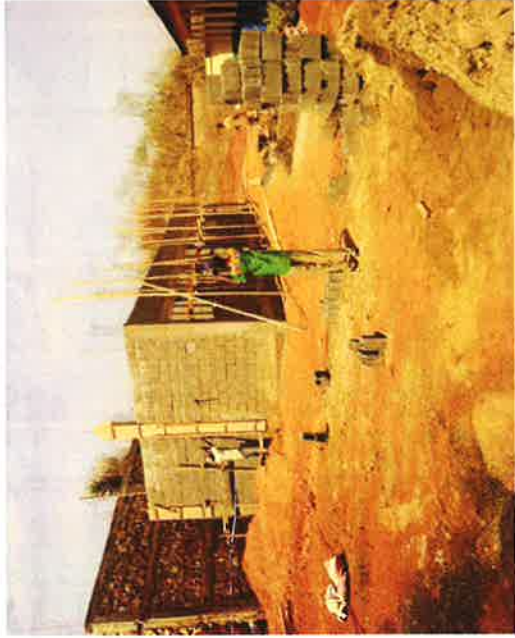
Construction of 2 classrooms in Rainbow College – Raising of walls
