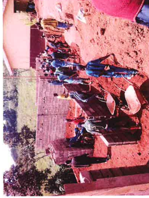
Construction of 2 classrooms in GHS Litieu – Community participation in filling of the foundation and leveling of the yard
